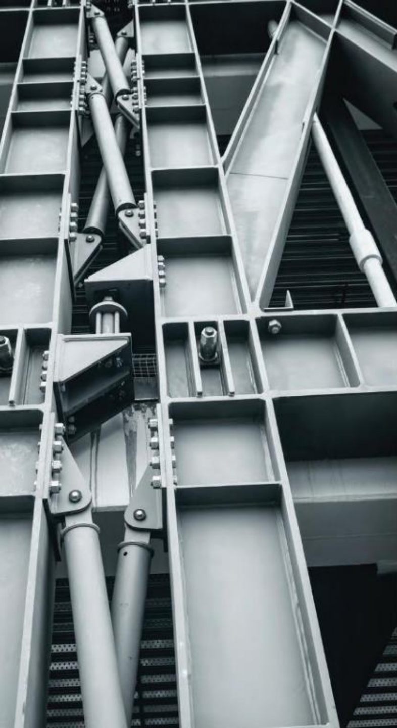
› Predrilled plate, structural bolts
