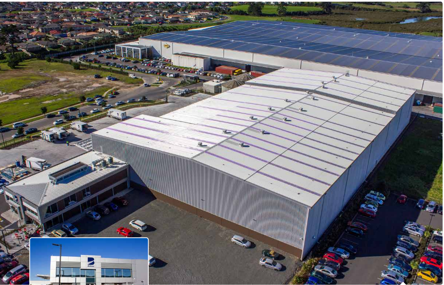
Bidvest NZ Ltd with Alsynite AITV 900 Ventilators
