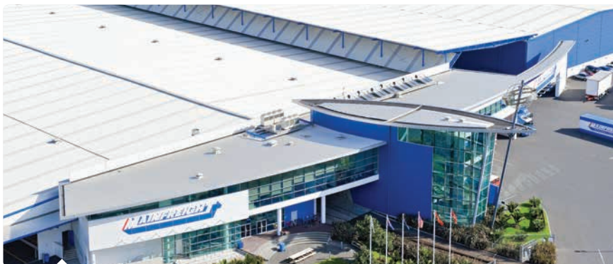
TOPGLASS® COLOUR: OPAL PROFILE: MAXISPAN® 2400 G/M 2
