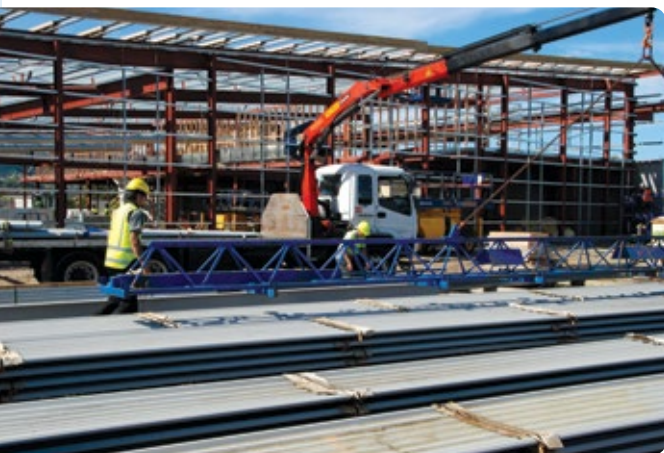
Steel & Tube and Premier Roofing at the Kapiti Landing Business Park's latest big-box retail development. Note the boom and spreader bar used to protect the long roofing lengths during lifting.
