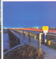
Hokitika Bridge, one of the longest in the country, totally supported with Steel & Tube product.
