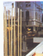
CP Reinforcing product at the Parliament Refurbishment Site.
