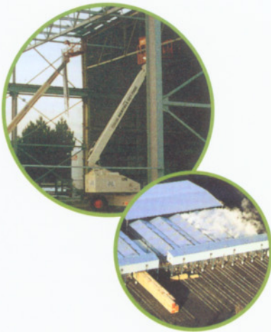
Dry kiln installation at Weldwood of Canada Ltd in Hinton, Alberta.
