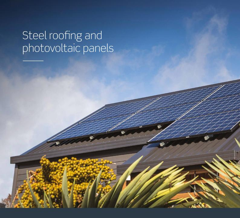
Framed photovoltaic (PV) panels can be successfully installed on COLORSTEEL® prepainted steel and ZINCALUME® steel roofs.
