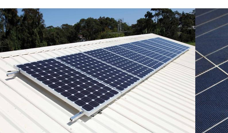
Also, consider using 0.55mm gauge COLORSTEEL® roofing if frequent roof traffic is anticipated. Any dents may need to be rectified to avoid water ponding, which is more likely to occur on low pitched roofs.
