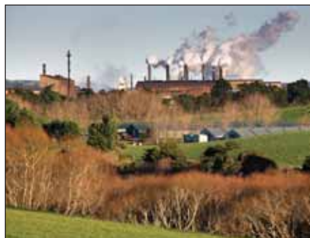
New Zealand Steel has invested considerable capital in its environmental management systems, in particular emission control, at the Glenbrook site.
